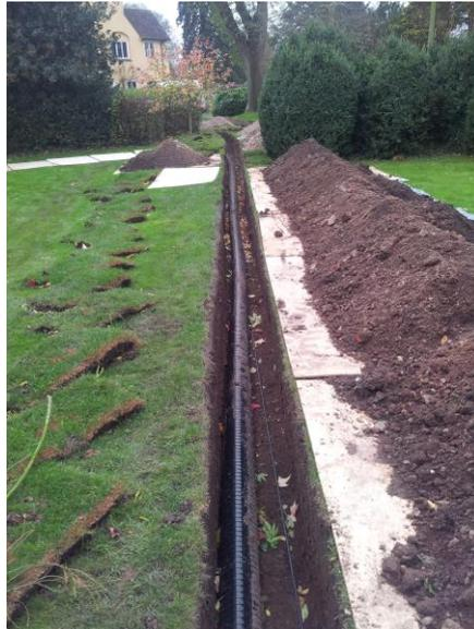
*Above and right: District pipe installed within a trench and a fan heater fitted within the greenhouse.*
