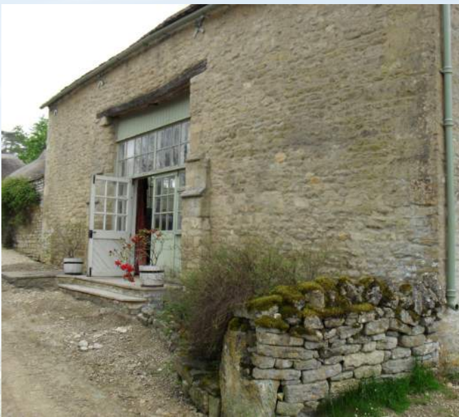
The third heated property at Lower House.
