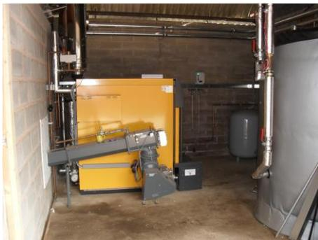
*The boiler, accumulator tank and expansion vessel within the plant room.*
