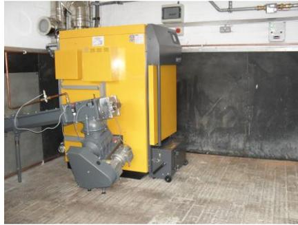
*The boiler and fuel store have been fitted within an existing stable block*
