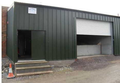
The new biomass building and fuel store
